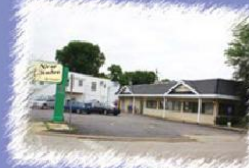
514 State Street. Dave & Cheryl purchased building from Tom & Mary Vavaroutos, March 2000
